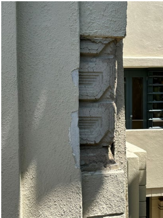
Photo 12 Exposed decorative knit block adjacent to south balcony, looking north
